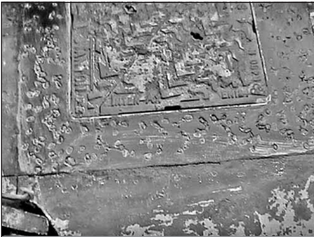
Fig. 9. Mastic asphalt reinstatement
